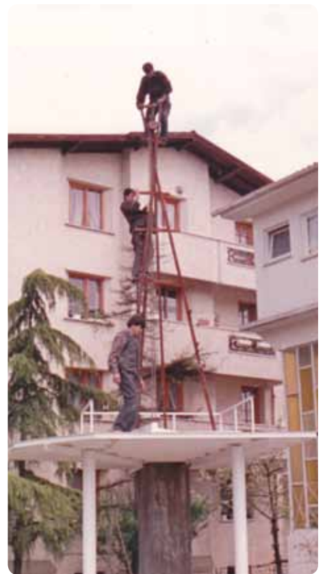
■ The mounting frame is being prepared
