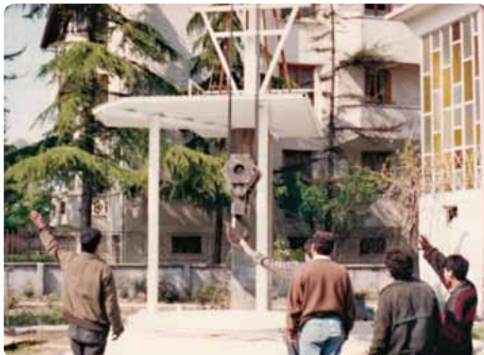
■ The crane lifts the dish in place
