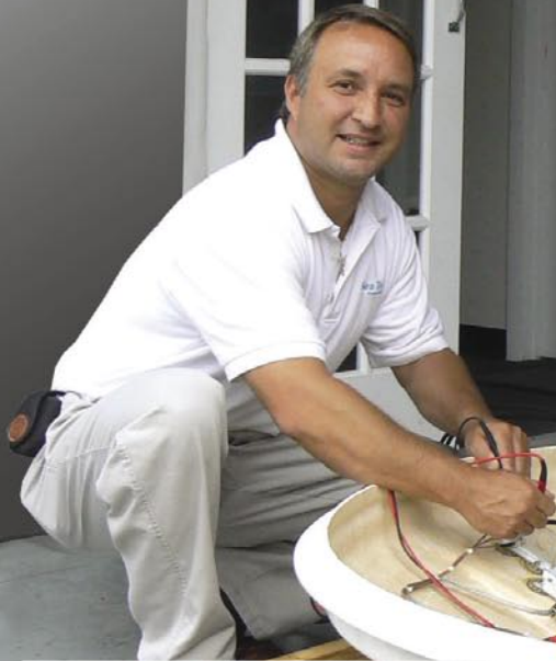
■ Steven Calice is also a Field Service Support Technician. Here we see him installing the new five-satellite system with DirecTV dish. The radome can be seen in the background and serves to protect the system on the yacht from weather and waves.
