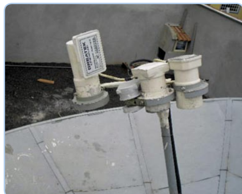
This is when it gets tricky: 4 C-band feeds are connected to each other
