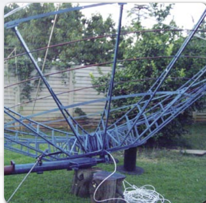
All of the support arms are now installed; next comes the installation of the aluminum reflector panels.
