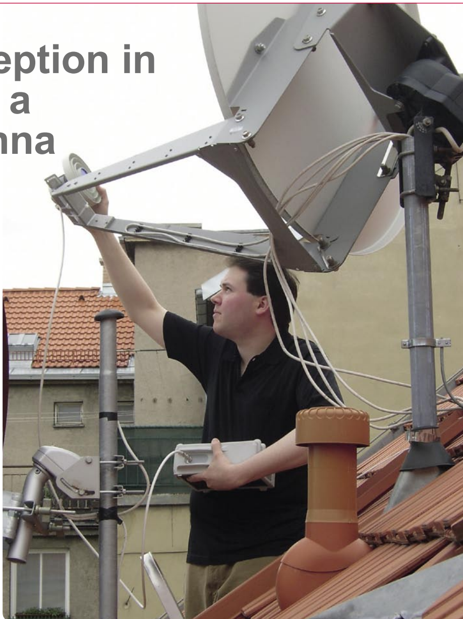
Thomas Haring adjusts a C-band feed on a 1.2-meter offset antenna while checking his progress with the help of the Prodig-5 signal analyzer also introduced in this issue |
